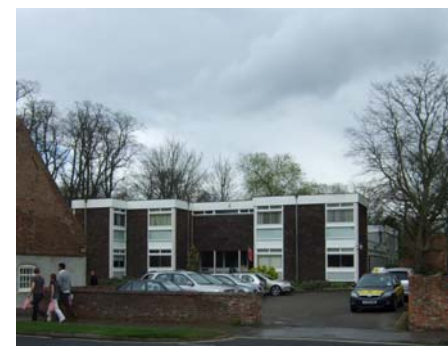
Plate 44 Unsympathetic building, east side of Main Street
