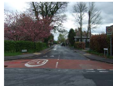
Plate 50 Excessive signage and road markings
